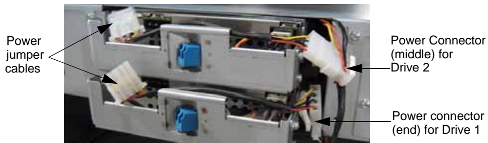
Figure F-1 Connecting the power jumper cables (LTO-4 drives pictured)
